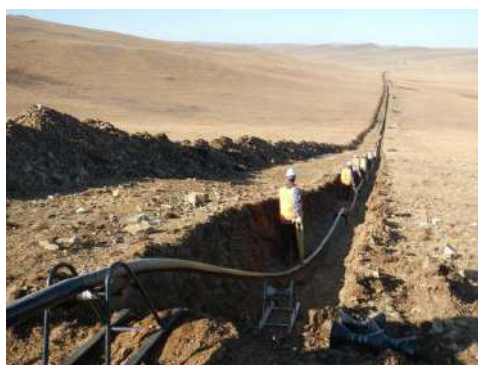
Source: Assessment team of Figure 2.11 Cable installing process
