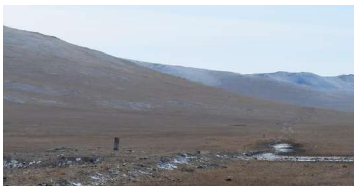
supplementary clarification of DEIA, 2016 Figure 2.12 After cable installation
