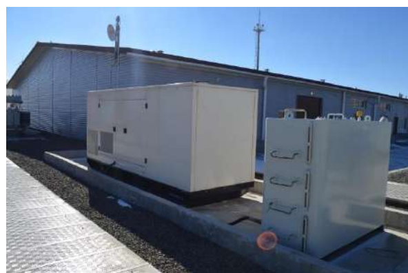
Figure 2.18 Diesel generator
