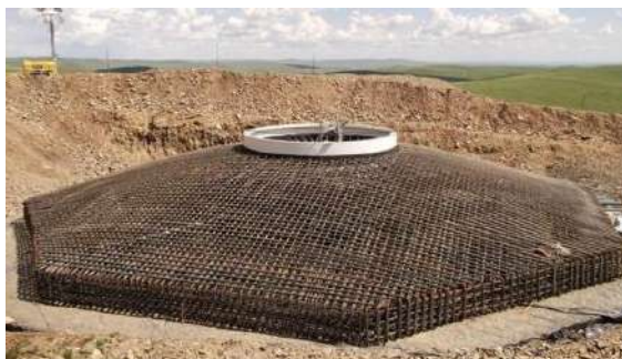
Figure 2.8 Foundation of wind turbine generator
