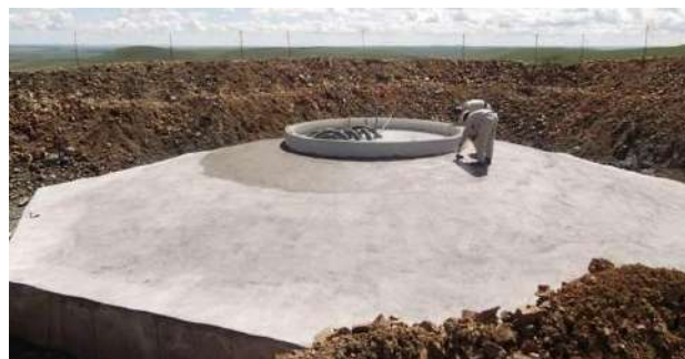
Figure 2.8 Foundation of wind turbine generator
