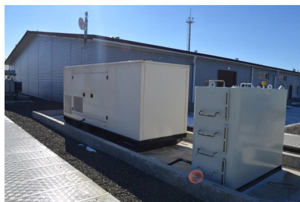
Figure 2.18 Diesel generator
