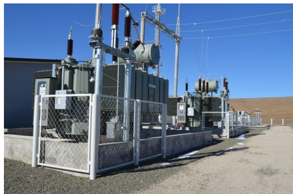
Figure 2.19 110/35 kV 50MVA - Transformer /from the front and left side, 2 pieces/
