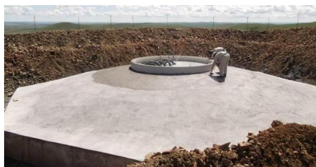
Figure 2.8 Foundation of wind turbine generator
