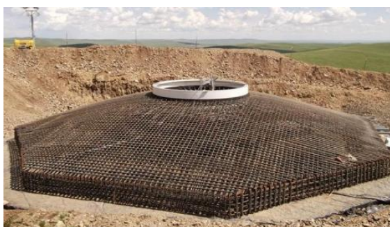
Figure 2.8 Foundation of wind turbine generator
