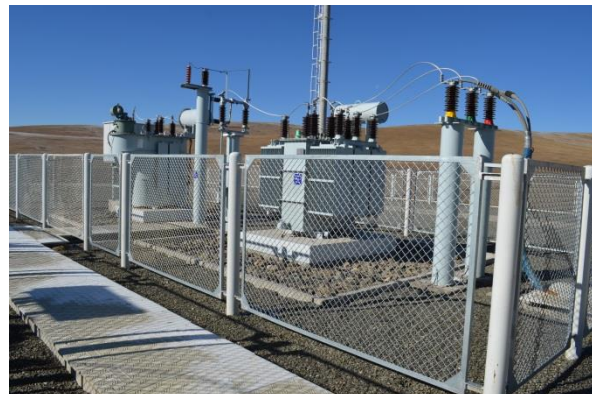
Figure 2.16 35kV electric arc dissipating coil
